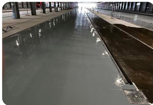
Autonivelante weberfloor PX TOTAL | Nave industrial
