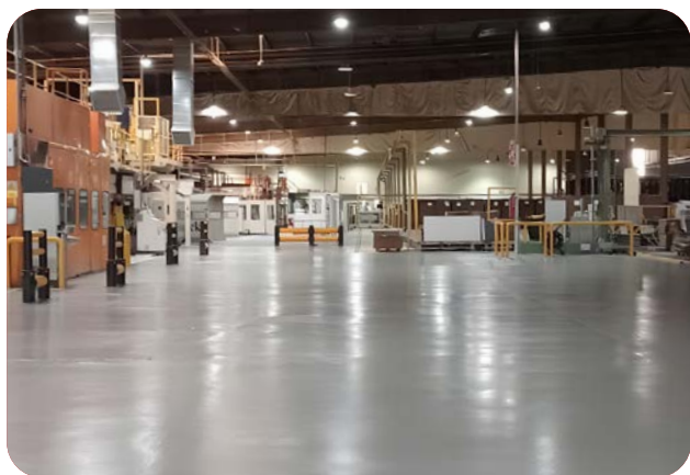
weberfloor PURLEVEL y PU INFINITY 2C | Nave industrial
