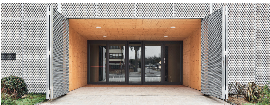
104/ Centro Cultural Torredembarra
